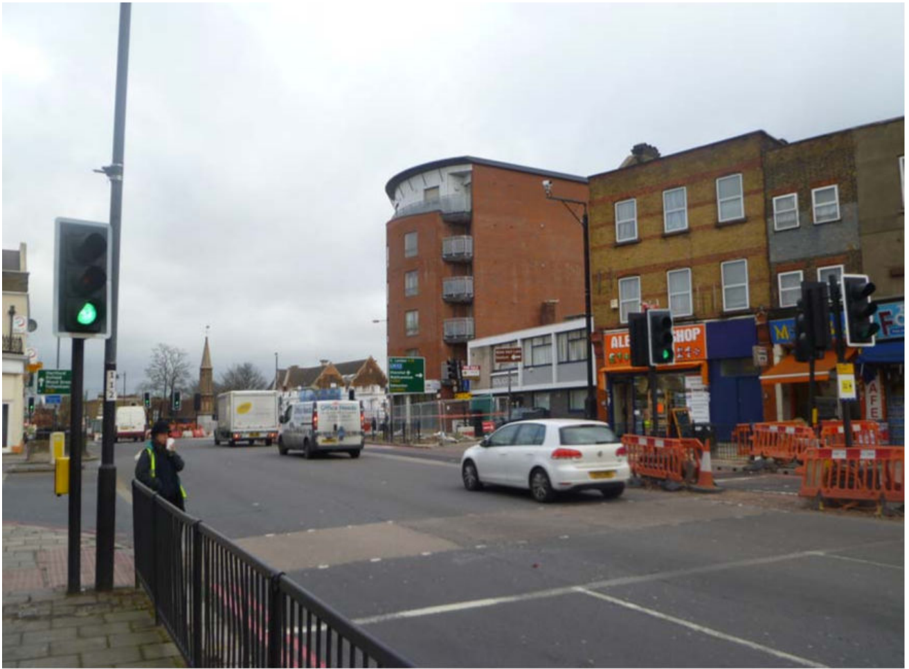
View from the High Road
